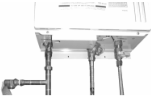
Pressure relief Valve HOT
